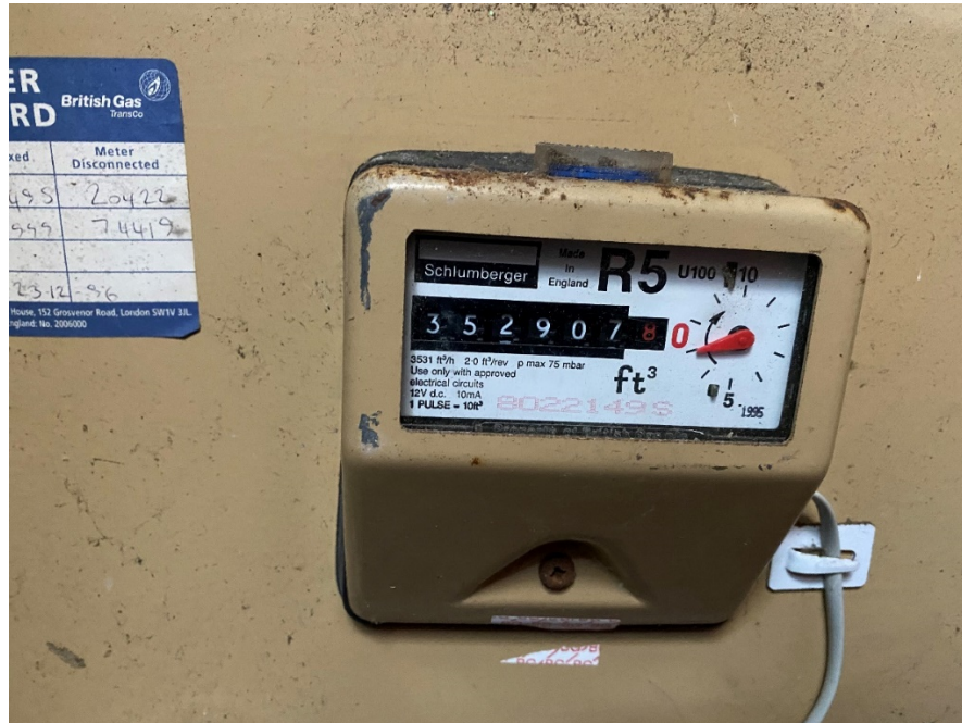
Fig 4 – Gas Meter
